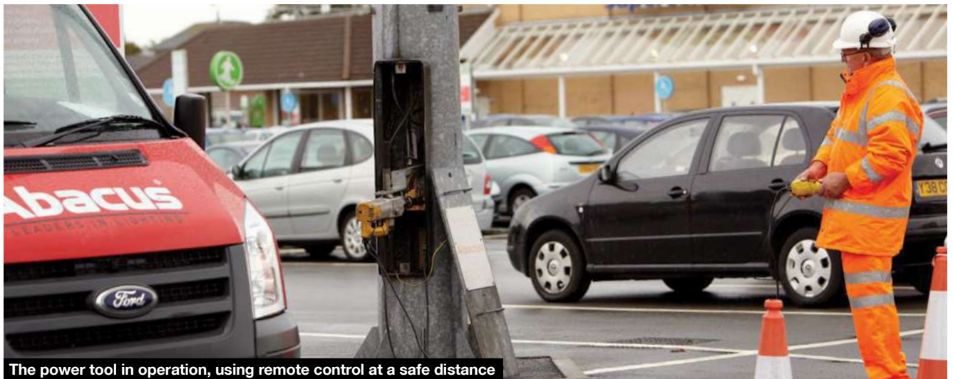
The power tool in operation, using remote control at a safe distance
